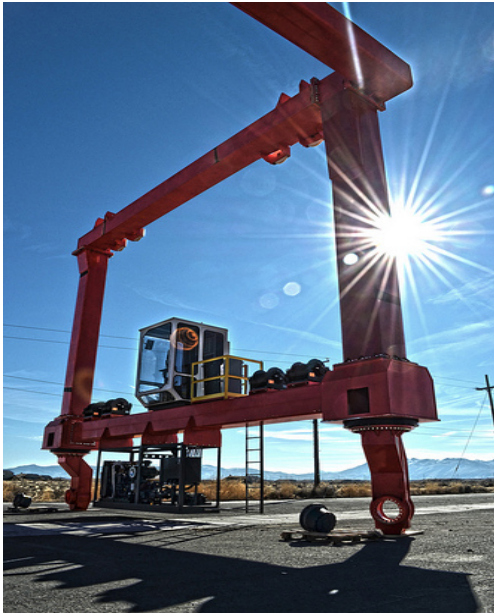
100-ton gantry crane nears completion at Sierra Army Depot.
